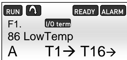
Figure 5.1-3, Low temperature alarm on the NXP panel
